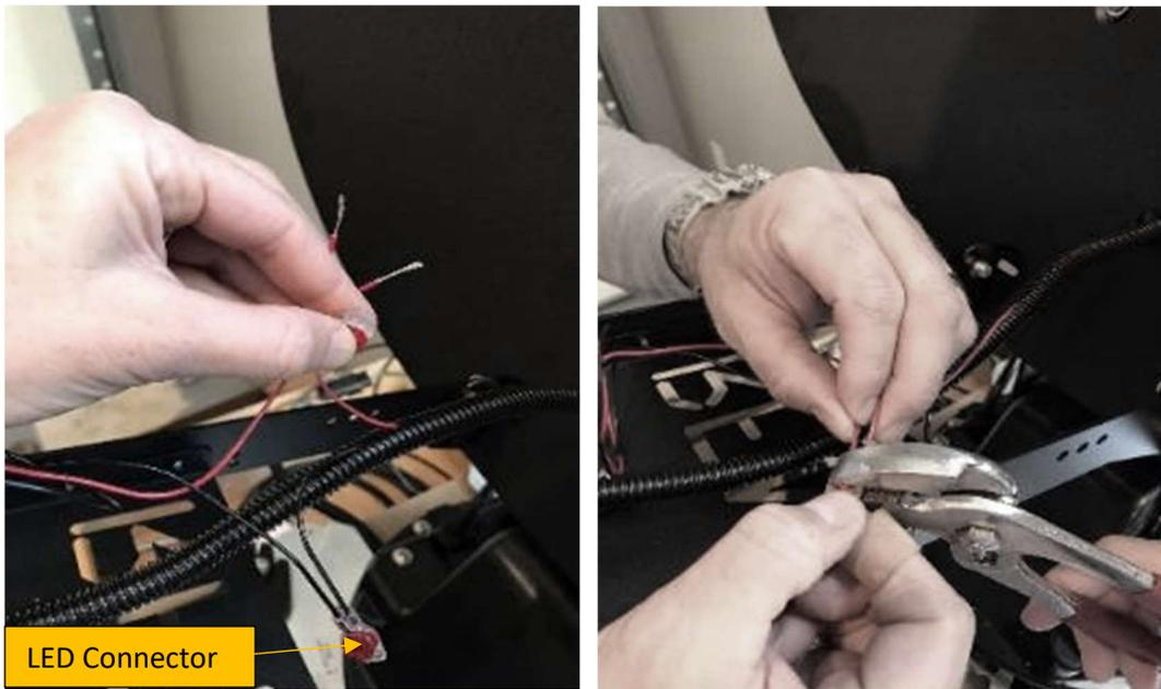
11. **Route** the Cable Loom down either side of the LNB Arm and secure with Cable Ties (provided).
