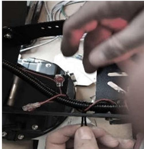
12. **Tuck** any excess Cable Loom back through the Reflector. Leave enough out to prevent binding.
